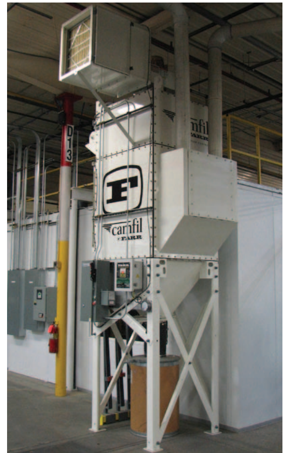
▲ One GS4 unit that helped Viracon transition from a wet to a dry process.
