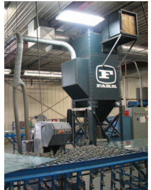
▲ A GS4 is installed at another trimming unit.
