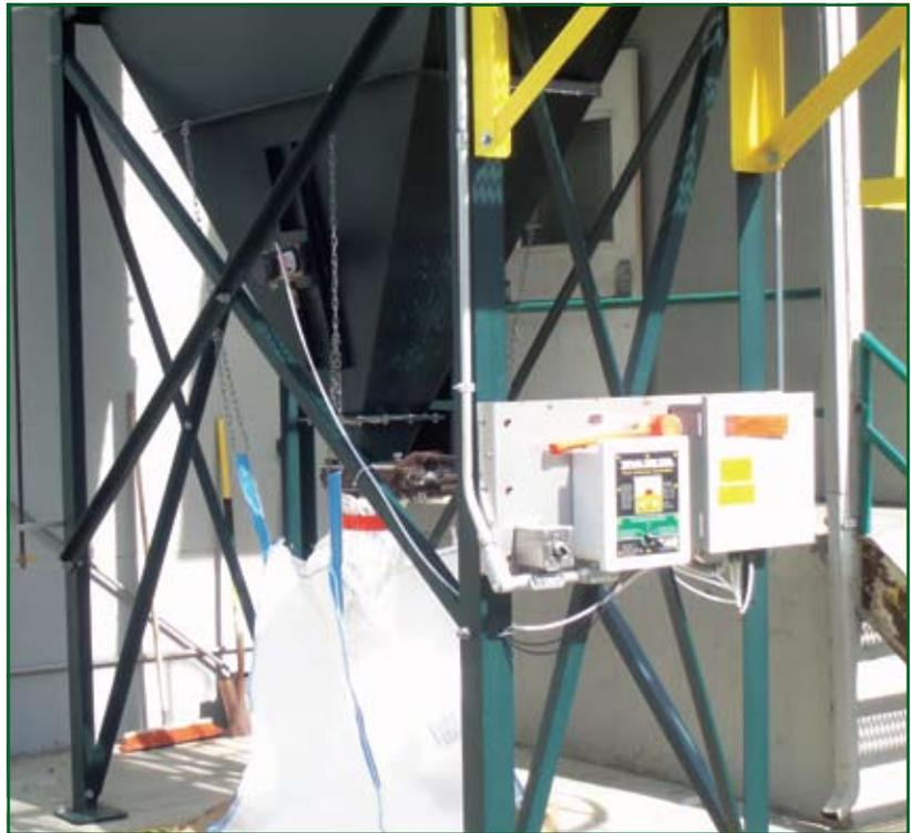
*This pyramid hopper features a special mounting bracket for a vibrator to aid in material flow.*
