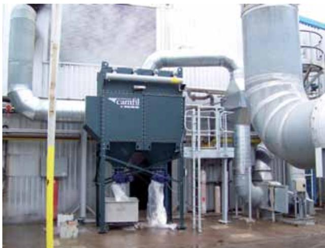
Entek chose Camfil Farr Gold Series® dust collectors ahead of strong competition because of the high efficiency and low pressure drop of the HemiPleat® filter cartridges. This together with the extremely quick filter change of the Gold Series and the low cost of replacement filters, compared to the DCE Sintamatic units, made the Gold Series the obvious choice, with payback being as little as one year.
