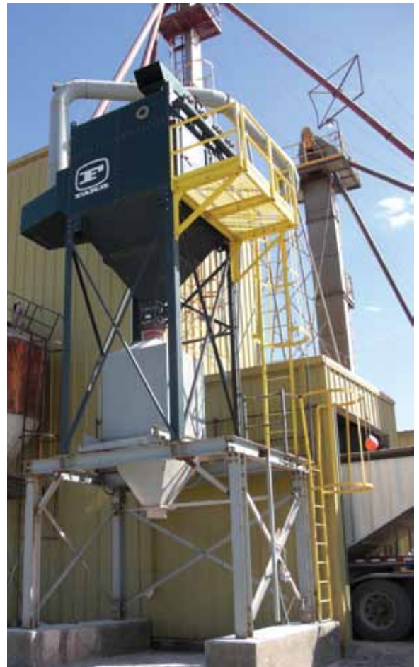
Up in the air GS16/12 collects the airborne product that is loaded into the semi trucks.
