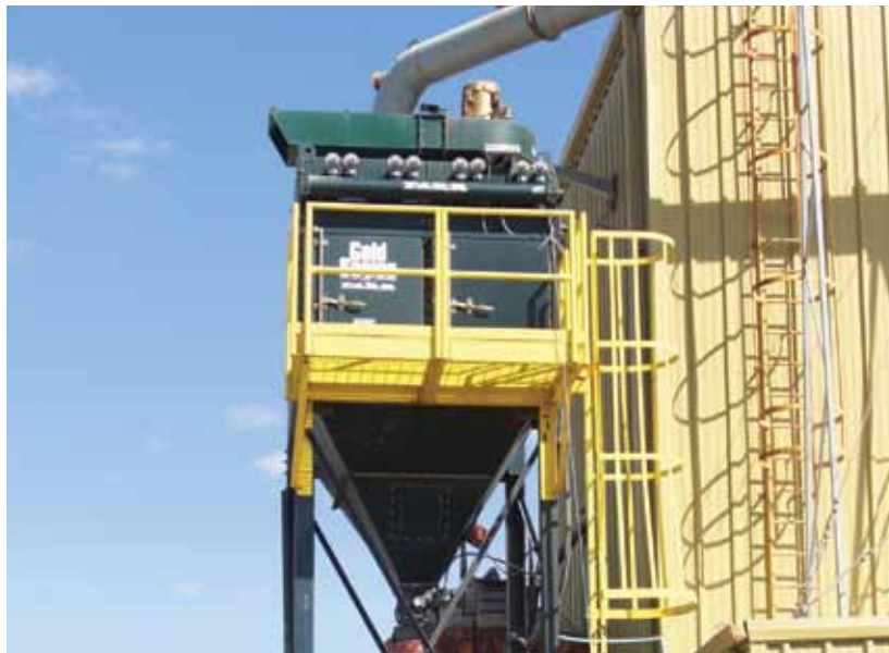
Gold Series® model GS16/12 replaced a cyclone, which used to emit product into the air.
