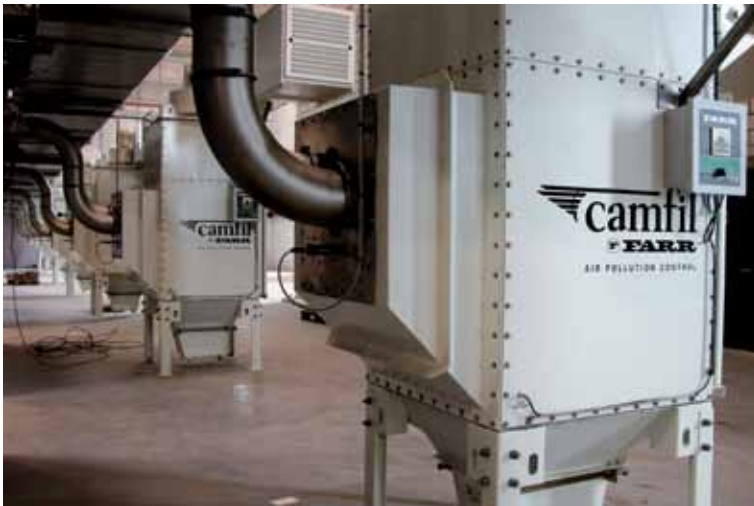
Farr Gold Series dust collectors on the production cells.
