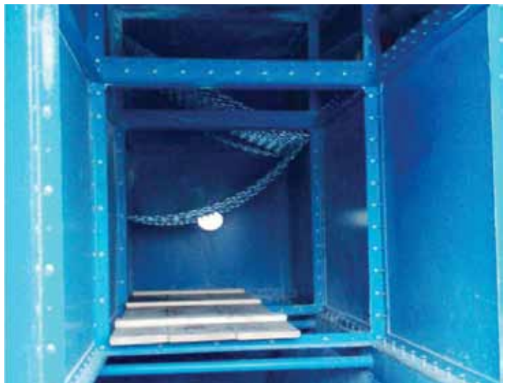
Inserted chains in drop out box.
