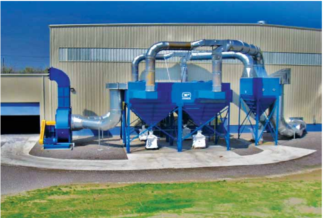
Completed solution for National Bronze & Metals, Inc. to meet strict EPA lead limits.
