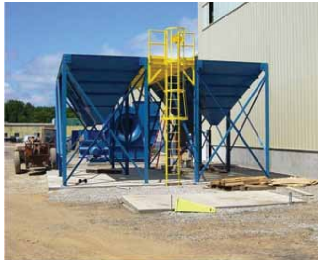
Installing the hoppers.
