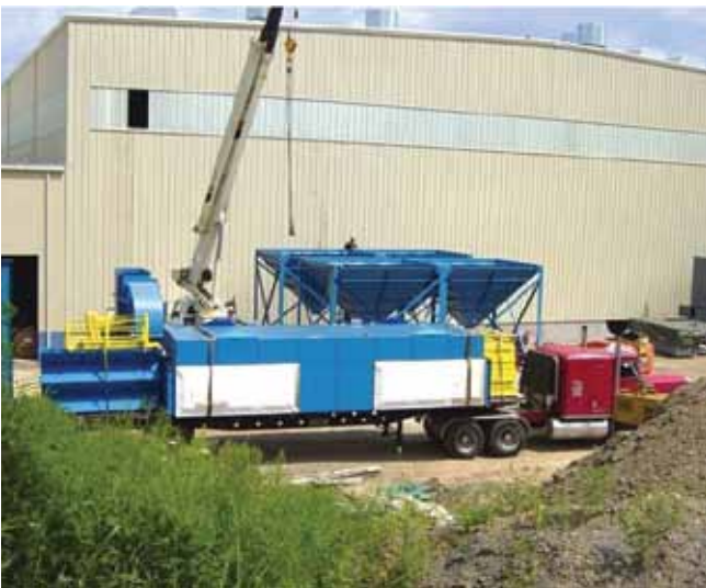
Setting the collector in place.
