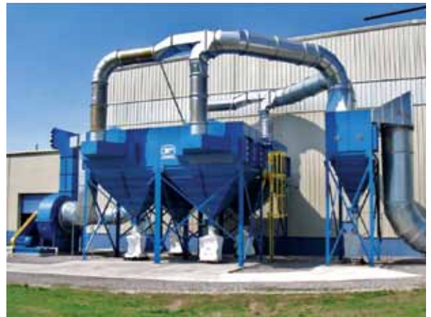
Gold Series model Tandem GS96 collecting fumes from metal processing.
