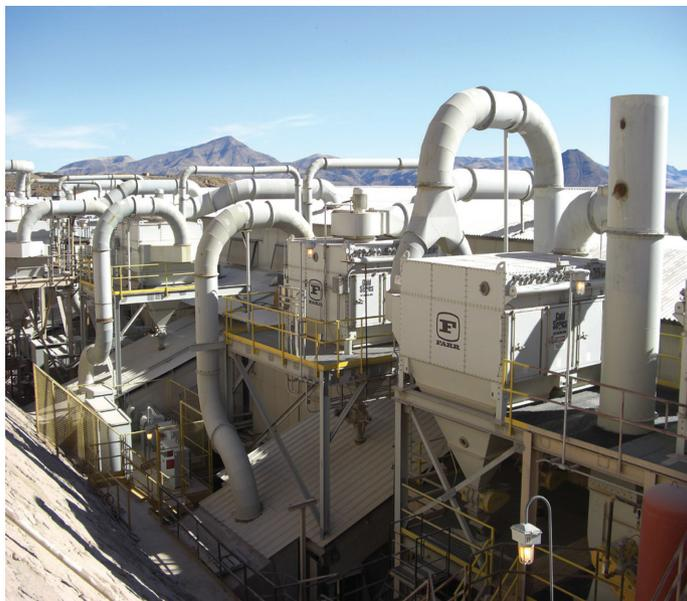
avoid problems of filter plugging due to moisture in the ore. The pleated filters are mounted vertically inside the collector, eliminating the dust blinding and premature failure that sometimes occur with horizontally installed filters.
