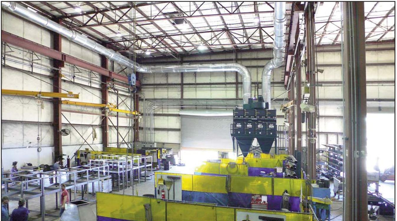
*Gold Series GS48 on Welding Fumes - Farr APC installs a Gold Series collector in its own welding shop.*
