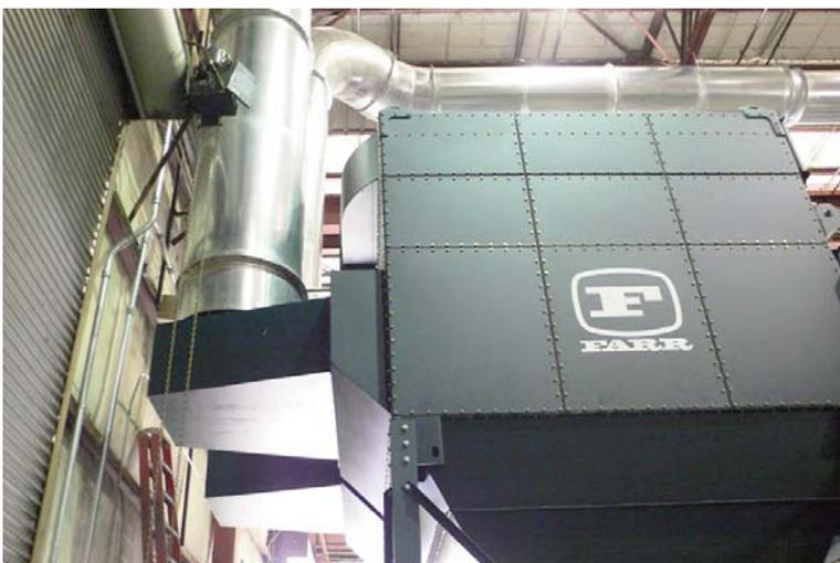
**Right Angle Inlets** (normally offered as abrasion resistant inlets) facilitate easy transition of airsteam into the collector.
