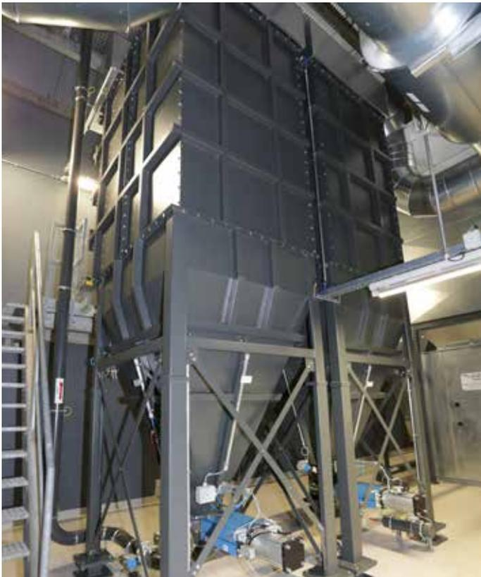
Four modular MF-ULTRA 194.3.1 units, each with 12.500m<sup>3</sup>/h volume for extraction of the milling machines with pneumatic dust and chips removal system
